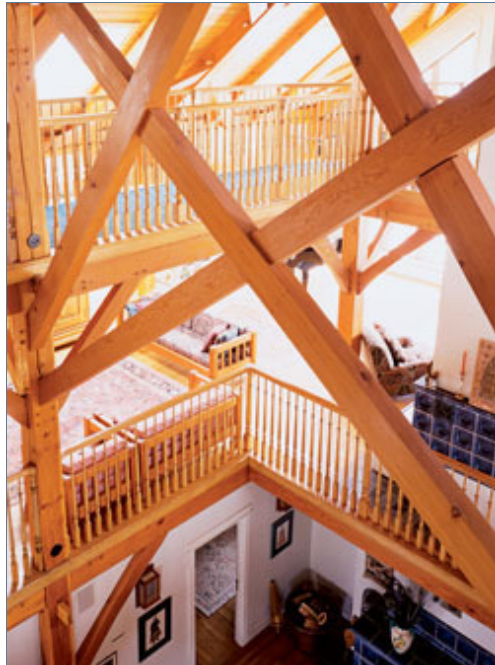
EXPOSED: X braces in a Nova Scotia residence.
