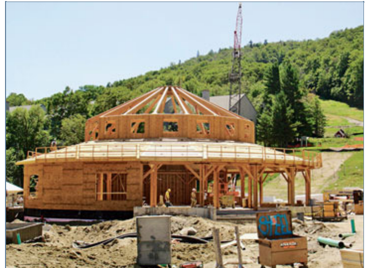
Courtesy Fire Tower
